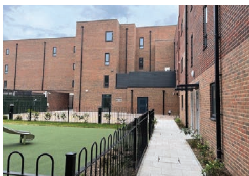
Above: Front and back at Lester House in Parsloes Avenue – our brand-new scheme in Barking and Dagenham.
